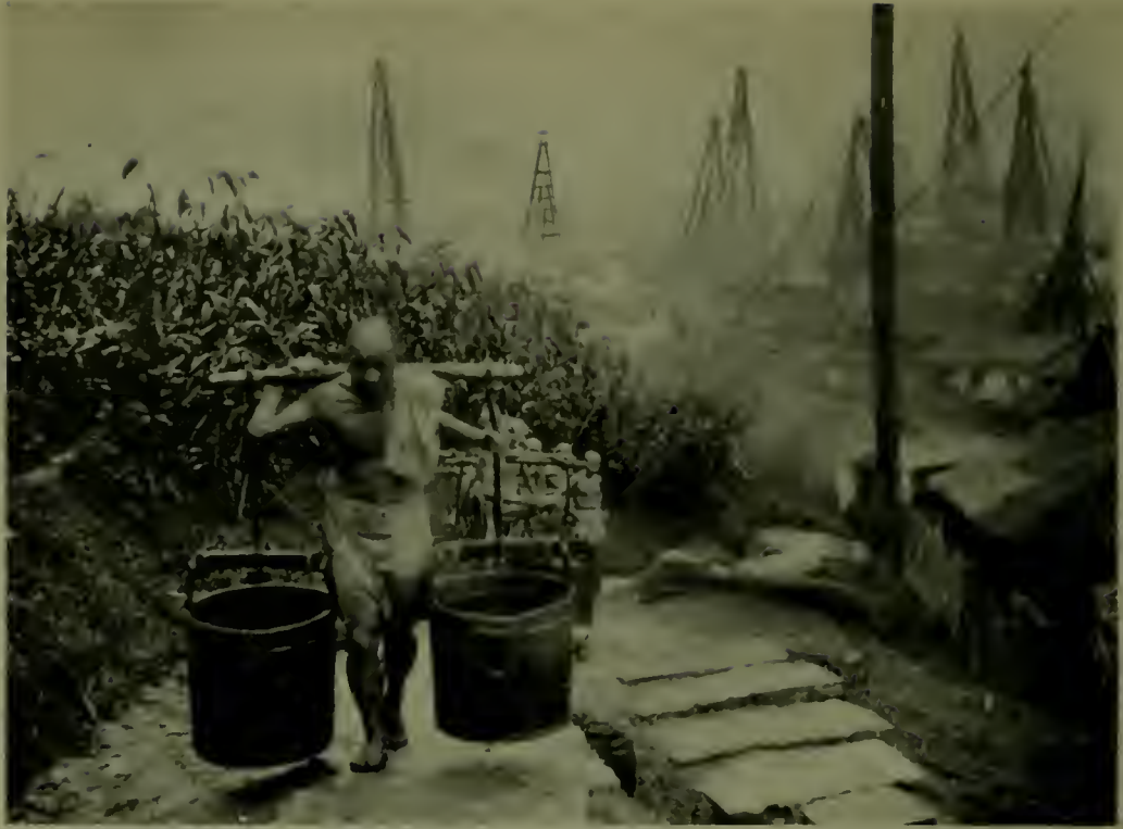
Long trains of coolies carry immense buckets of water from near-by ponds and similar unsavory sources of supply to turn into brine the rock bottoms of the salt-wells, the derricks of which punctuate the sky line of the Tzuliuching region
